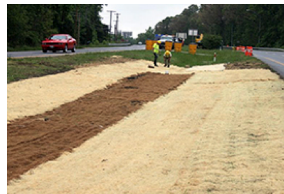
Figure 4.4-4 Linear Bio-swale (Source MDSHA)
