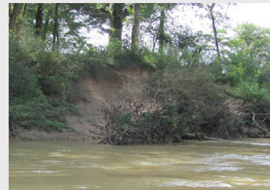
Figure 2.2-7 Chatahoochee River bank erosion caused by fallen tree undermined by scouring in high flows Photo: CRNRA, National Park Service, 9/5/15)
