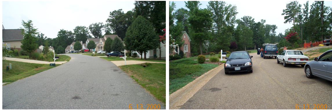
Figure 3.3-17 Narrow streets reduce impervious cover area.
